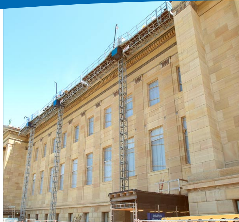
KPM-8 platforms supporting restoration work.
