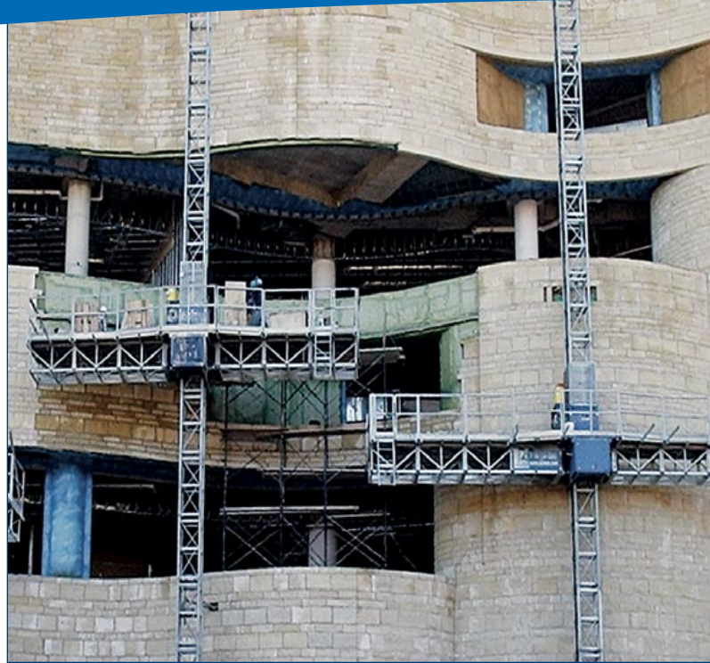
Multiple KPM-8 platforms at work on a large-scale masonry project.
