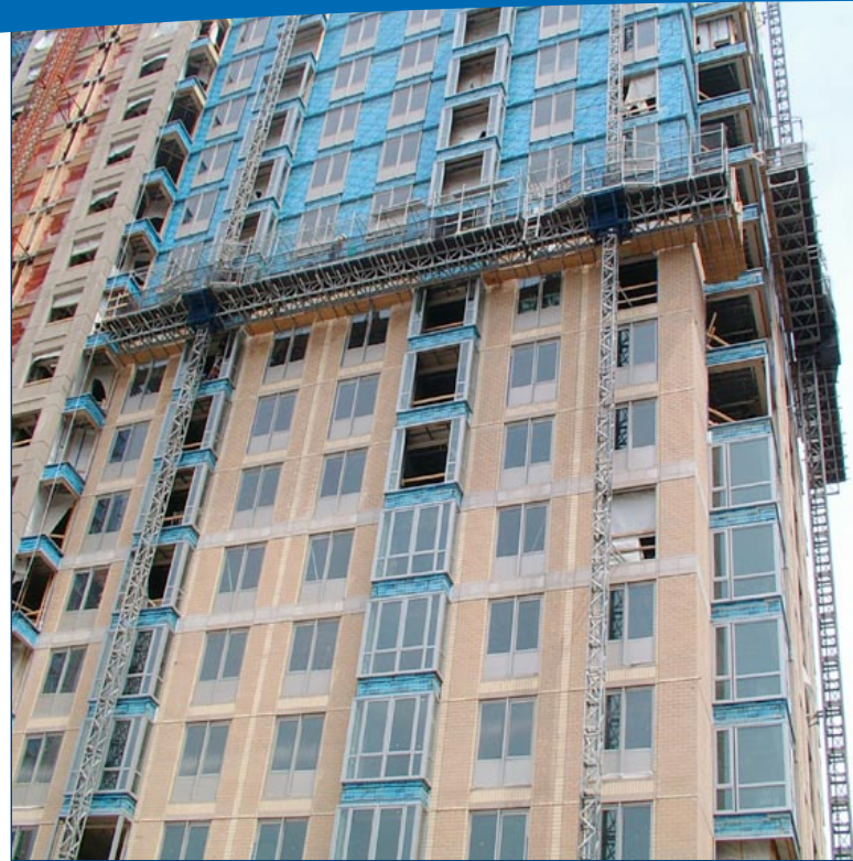
KLIMERLITE provides complete project access for multiple trades.
